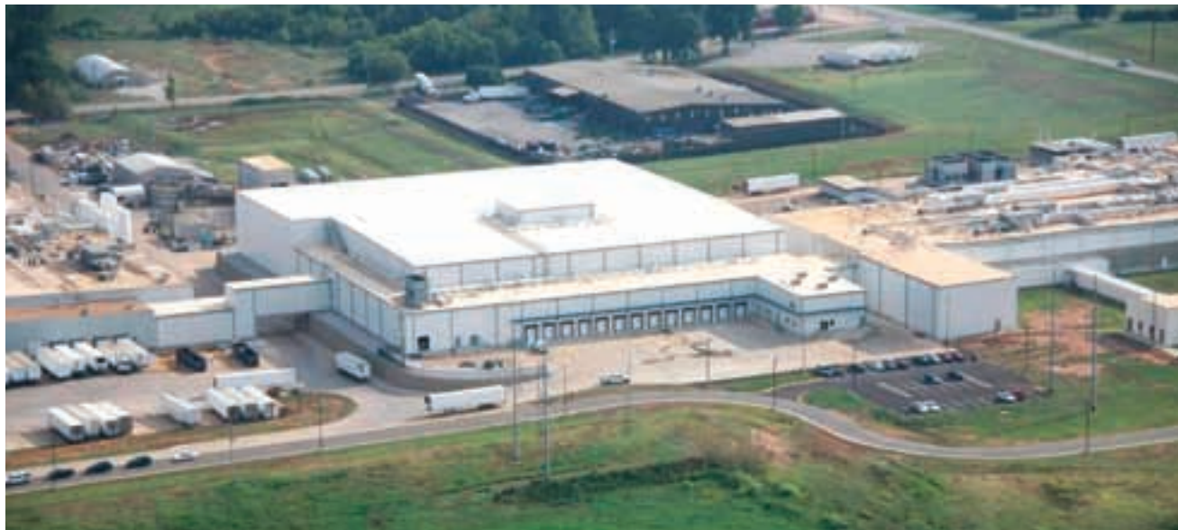
After Wayne Farms LLC, Oakwood, Ga., completed significant processing expansions at its Decatur, Ala. campus it targeted the plant's complicated distribution network. (Photo courtesy of Primus Builders)
